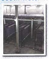
This plant was built in 2012 to treat water from Lake Alan Henry. The water from Lake Alan Henry is treated by passing through membrane filters that remove small particles and impurities.
